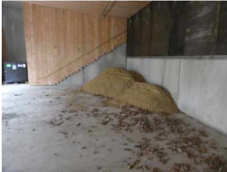
1-3: Construction of a bullet stop housing, filling
