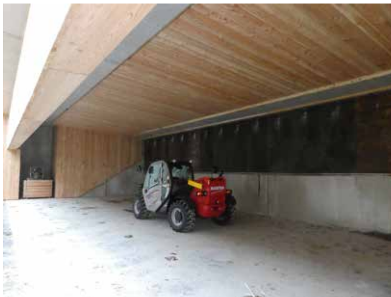
1-1: Construction of a bullet stop housing, overview
