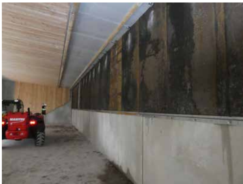
1-2: Construction of a bullet stop housing, rear wall, roof, ceiling
